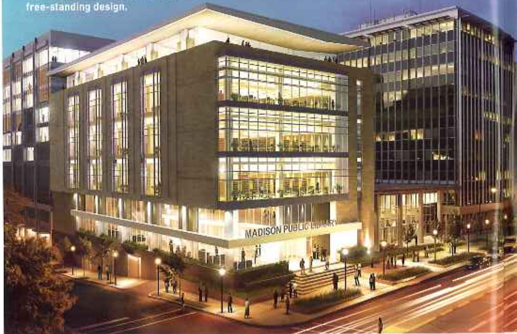
Lighting up West Wash: Fiore-Irgens' free-standing design.
