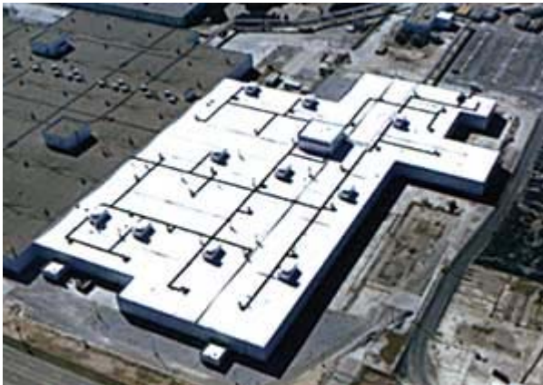
GM plant aerial view Courtesy of Ghafari Associates, Dearborn, Mich.
